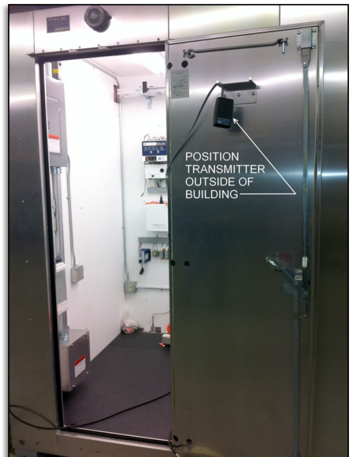
Figure 4 - Suggested Location for Transmitter
